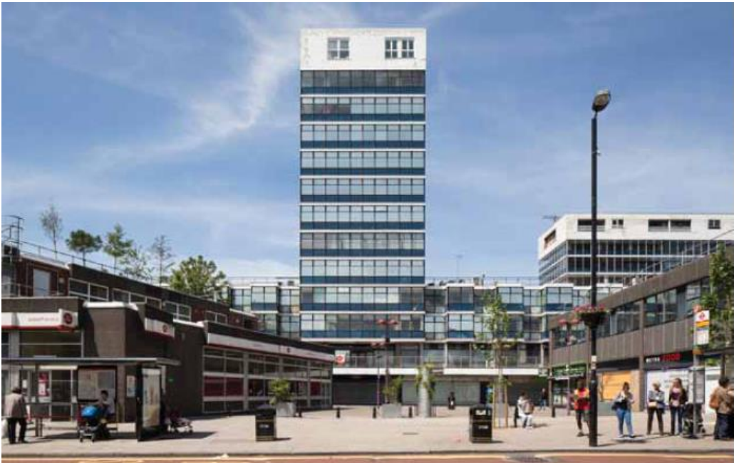
Existing building and Archway Town Square from MacDonald Road Page 198
