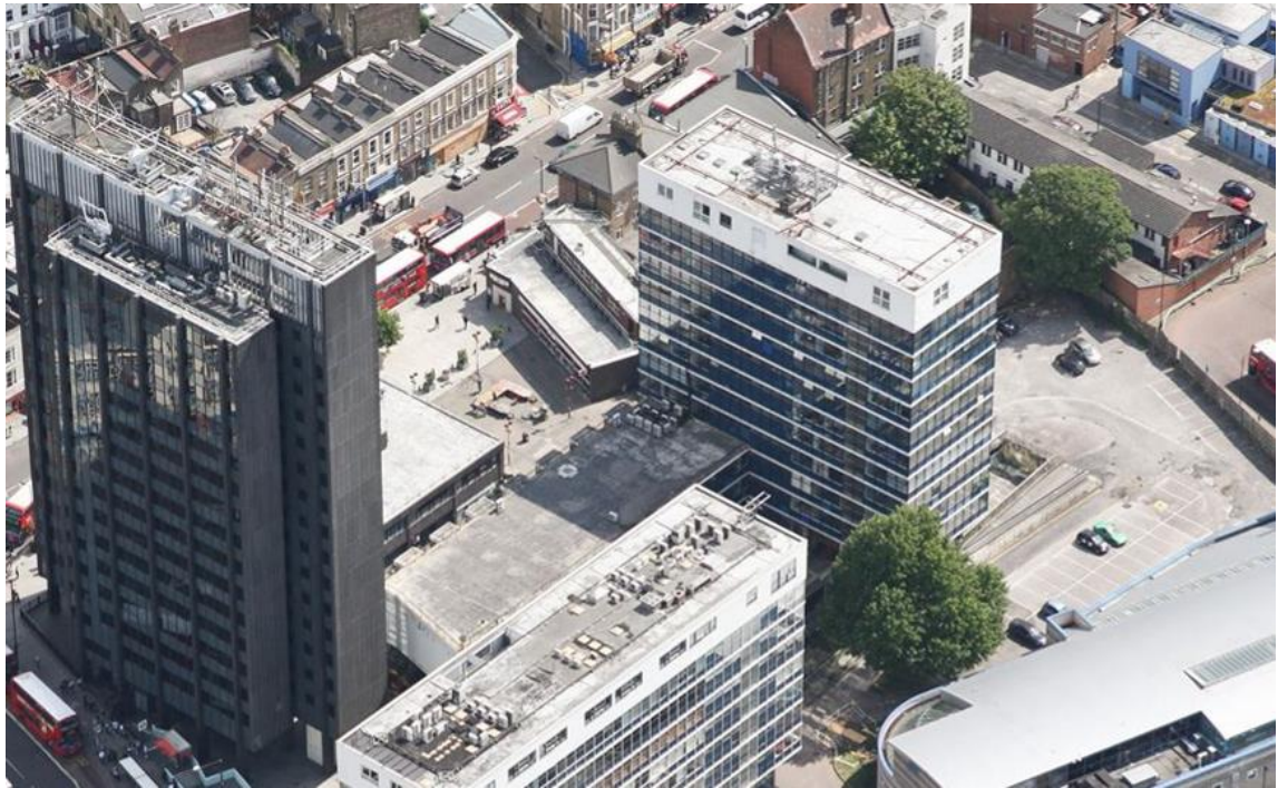
Existing building (looking west)
