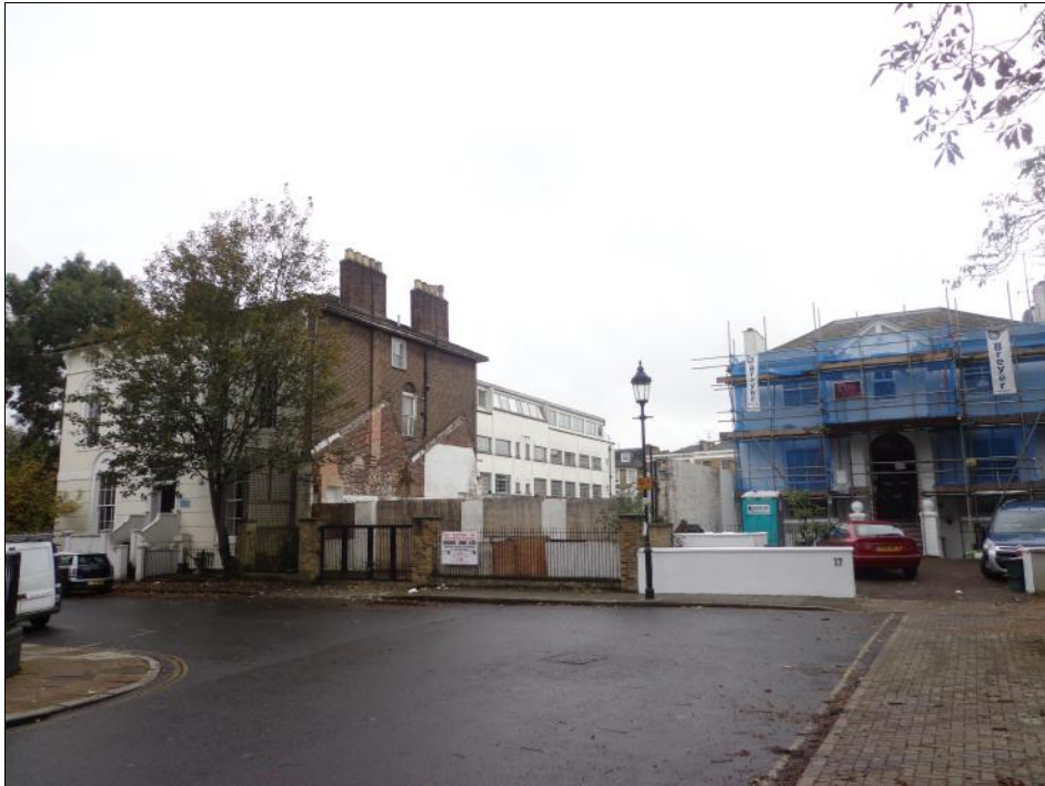
Image 2: View of application site from Barnsbury Square following demolition.
