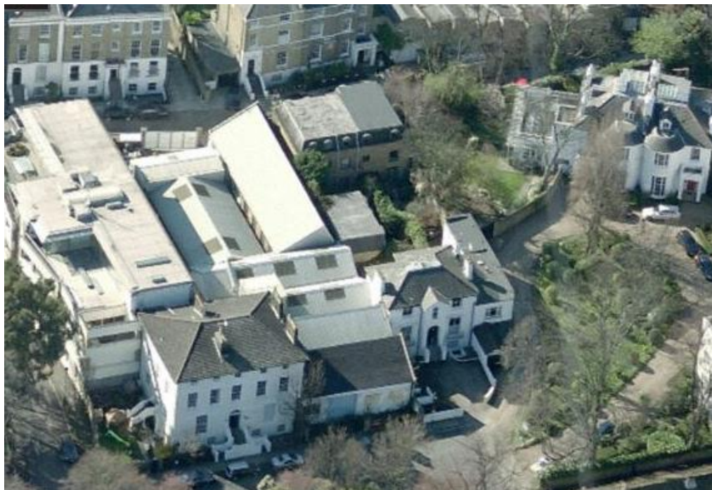
Image 1: Site prior to demolition
