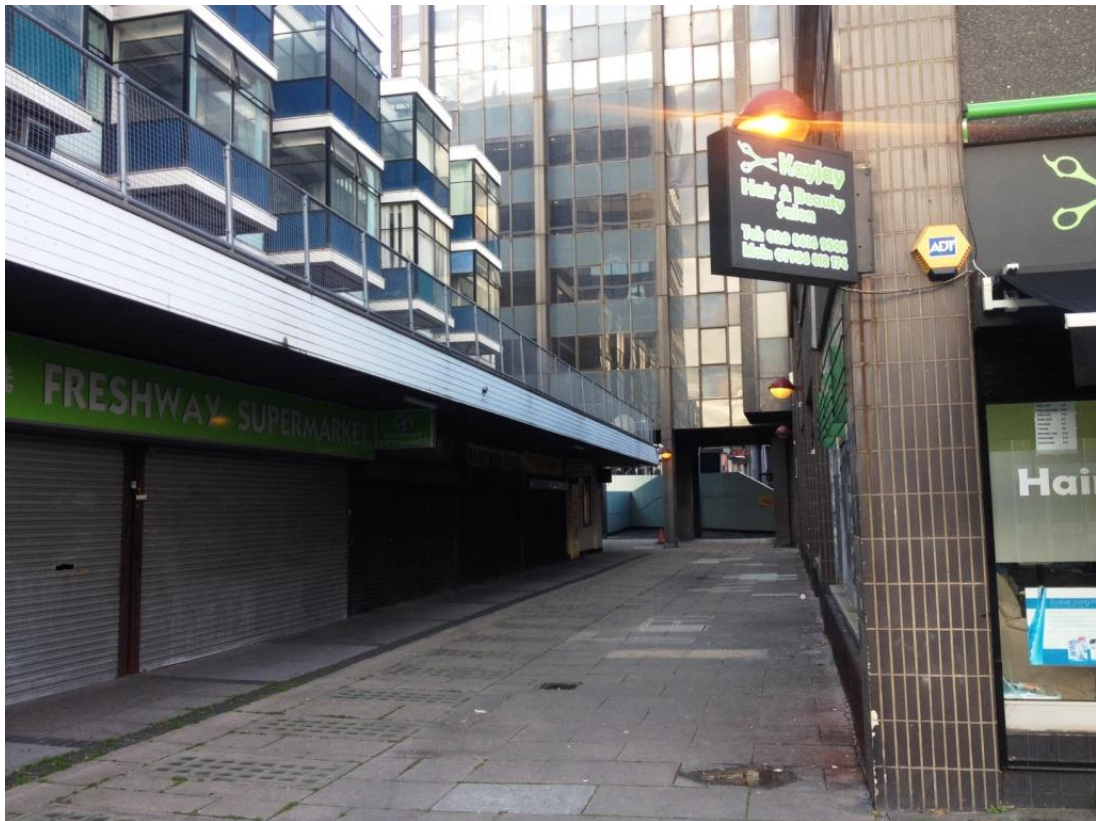
Existing shopfronts at the base of Hill House and pedestrian route to Holloway Road
